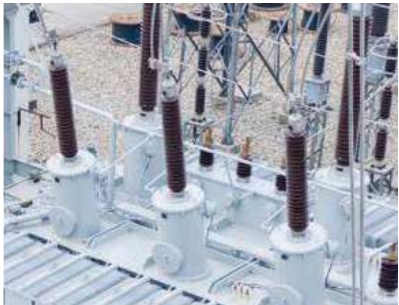
Fig.: High voltage transformer bushing
